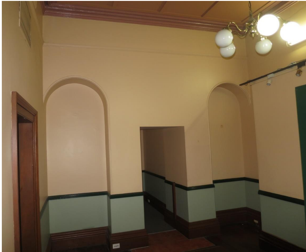
Figure 54 – the original dining room G.05 on the ground floor. The niches, skirting and cornice are original, but the central fireplace has been turned into a doorway to the former strong room. The chimney rises over the left niche.
