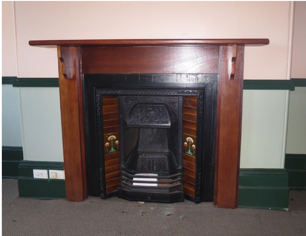
Figure 57 – the cast iron coal grates and their Art Nouveau tiles in rooms F.02 and F.04 are typical of 1910. They may have been installed after a late twentieth-century theft, rather than an early change. The hearth is bare sandstone under the carpet. The timber mantelpieces in these rooms are inappropriate and should be replaced with late Victorian style marble. The chair rails should be removed. NBRSArchitecture February 2017.
