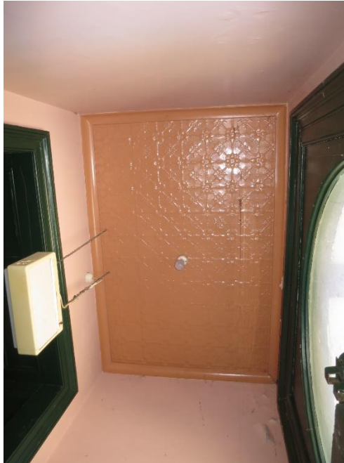
Figure 45 – pressed metal ceiling in G.01, (probably Federation period) and original joinery to the fenestration.
