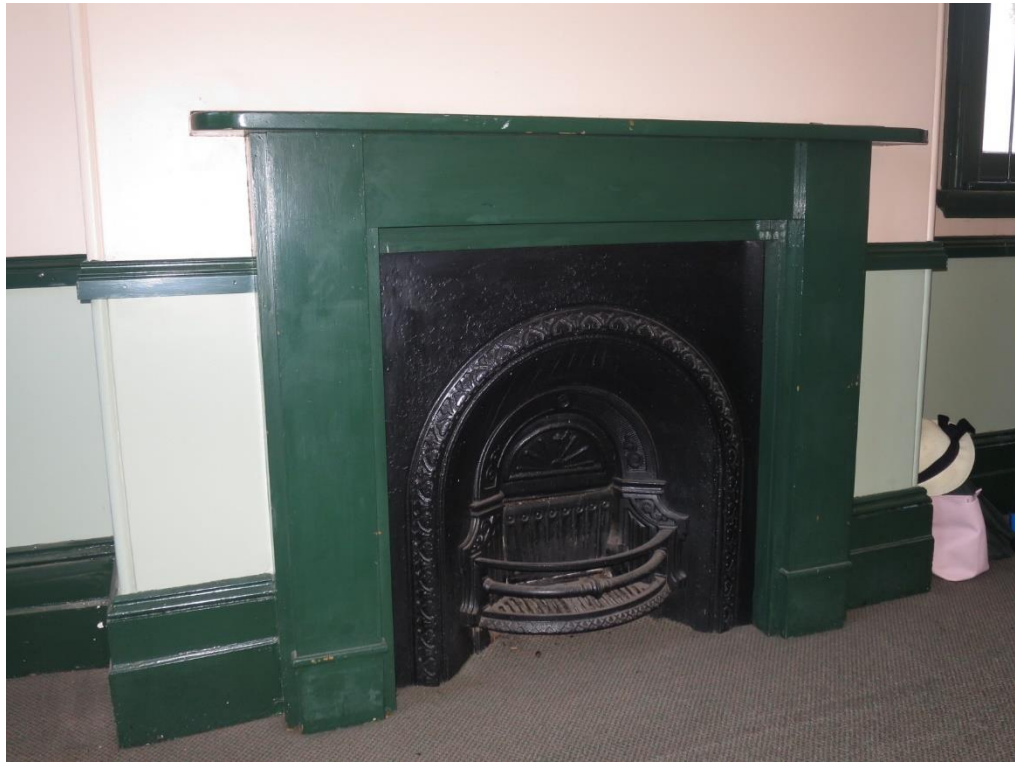
Figure 51 — likely original cast iron coal grate in G.03. the timber mantelpiece is recent and should be replaced with a Victorian design in marble. NBRSArchitecture February 2017.
