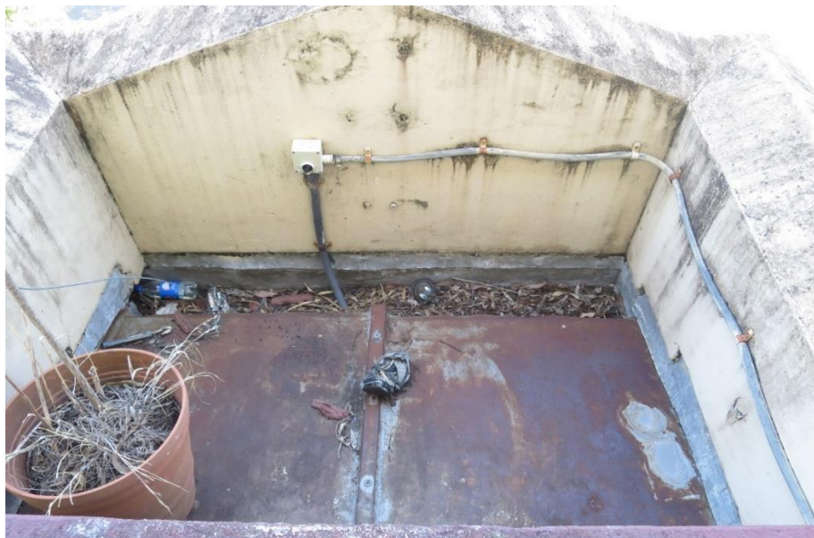
Figure 44 – roof and box gutter over the bank entry porch showing raised galvanised steel roof draining into a sump. NBRSArchitecture February 2017.
