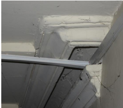
Figure 61 — a section of original whole cornice in the stair hall G.04. This is a good model for cornices in the former residential rooms that need to be reconstructed.
