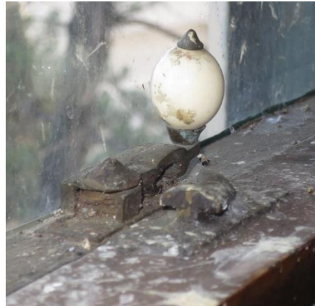
Figure 62 — an original brass and porcelain window catch that is a model for missing window fixtures. NBRSArchitecture February 2017.
