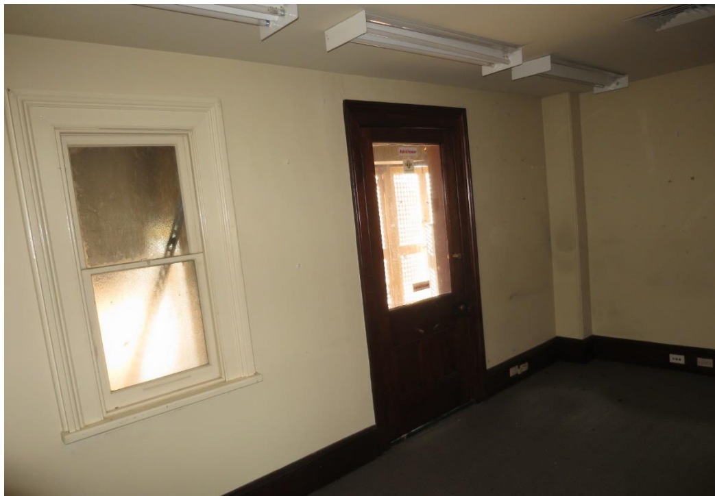
Figure 60 – Room 1.06m showing the original door that leads onto the rear verandah from the former bedroom, and the former bathroom window. There are two doors from the hall leading into this combined space. The low ceiling hides the air-conditioning distribution system. This door seen here has the only original lock and knob, apart from the entry doors. NBRSArchitecture February 2017.
