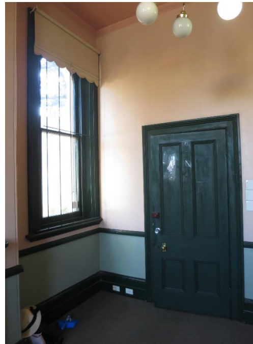
Figure 50 – original door and side elevation window in G.03 to be replicated in the conservation works.
