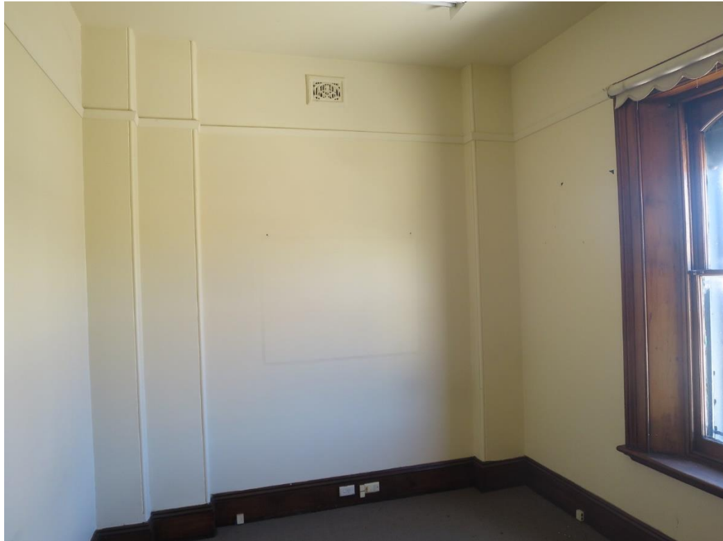
Figure 59 – Room 1.05 is a former bedroom with original door, skirting, window and staff moulds. The former chimney serving room G.05 rises on the left. NBRSArchitecture February 2017.
