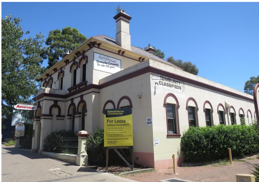
Figure 42 – southerly view showing the single-storey extension in the foreground that should be removed from the original building. NBRSArchitecture February 2017.
